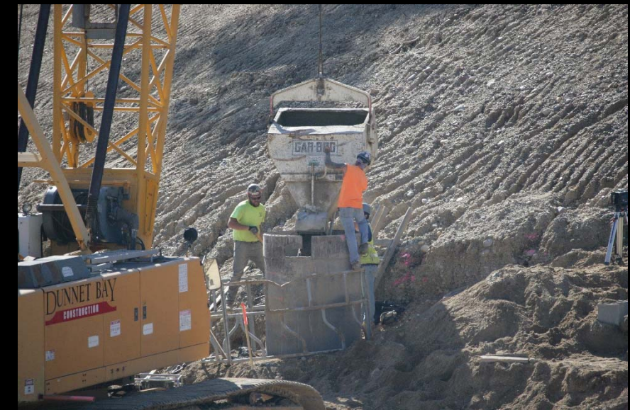
The contractor pours concrete for the retaining wall near Forest Drive on the LMP B-2 contract
