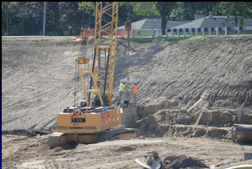
The contractor pours concrete for the retaining wall near Forest Drive on the LMP B-2 contract
